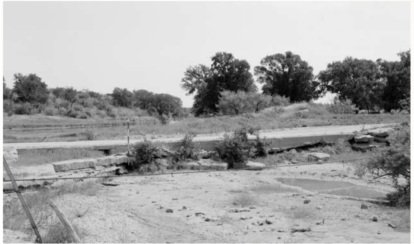
THIS 1989 PHOTO is of a bridge built from 1936-41 as part of a Works Progress Administration (WPA) project in Coleman County, Texas. Many Americans saw such projects as helpful, without considering their high cost and the corruption that plagued the program.
